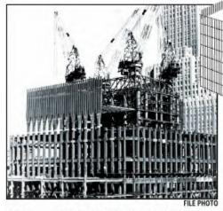
Steel assemblies hoisted during construction in May 1969. exterior wall
