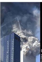
This photograph shows the south tower just as it is collapsing. It is evident that the building is falling over to the left. The North Tower collapsed directly downwards, on top of itself. The same mechanism of failure, the combination of impact and subsequent fire damage, is the likely cause of failure of both towers. However, it is possible that a storey on only one side of the South Tower initially collapsed, resulting in the "skewed" failure of the entire tower.
